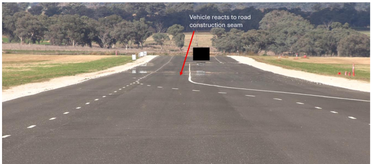
Figure 26: Example of the test track's tarmac construction seam
